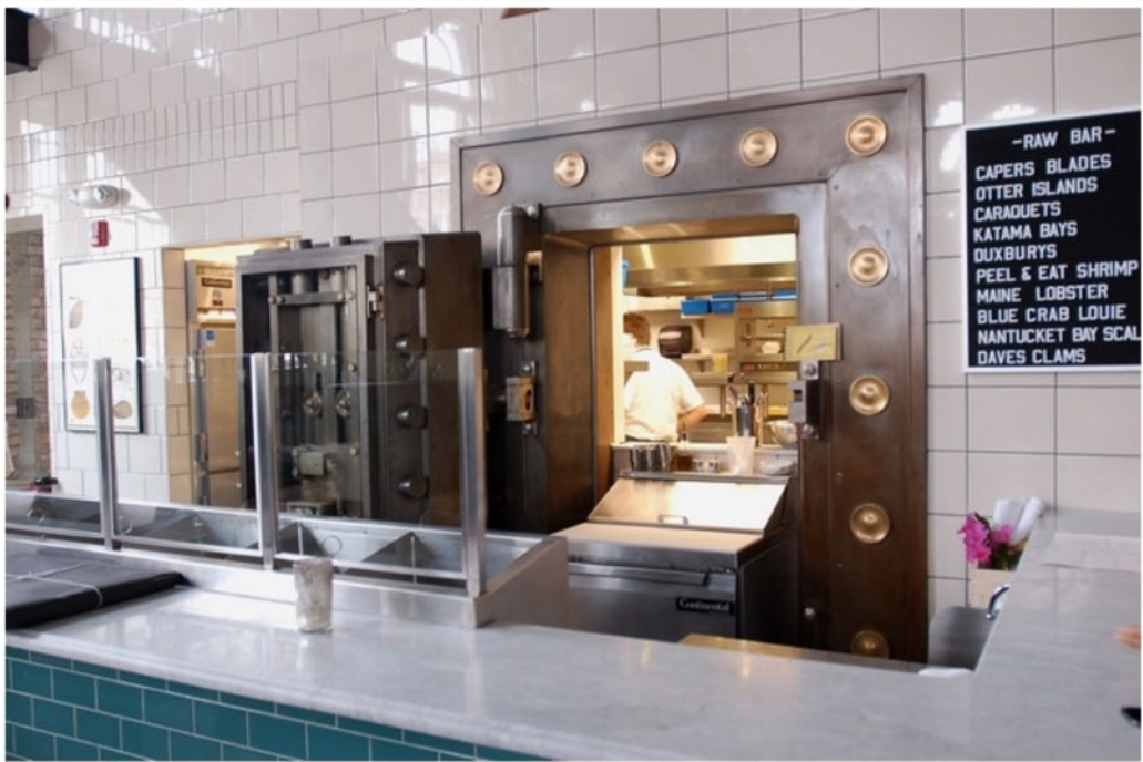
One major challenge in renovating the bank was deciding how to handle its massive safe, which ultimately was chopped up and its main part reused as a window into the kitchen.
